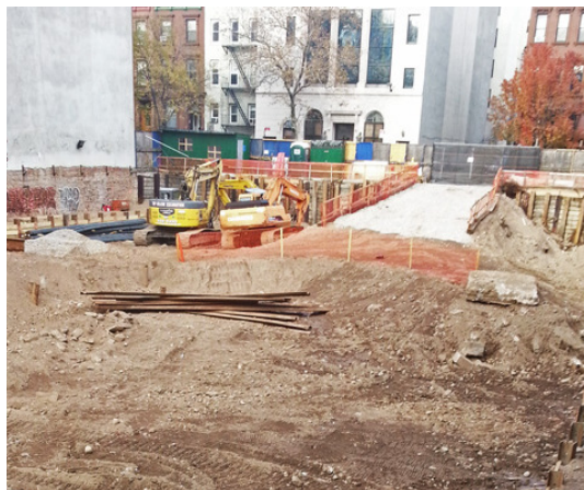
Construction underway 5-15 West 125 th Street
