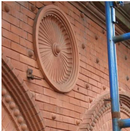
Corn Exchange Building Rehabilitation East 125 th Street & Park Avenue
